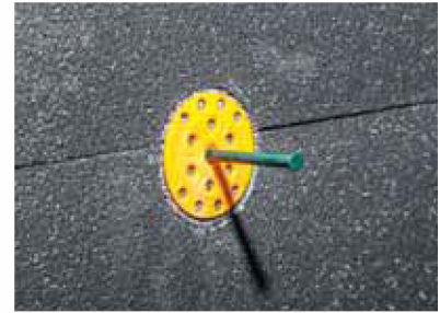
Figure 3 Wall plugs are placed in the holes, and nails are completely driven.
