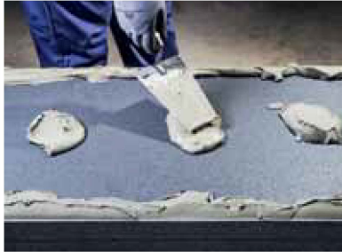
Figure 2 If there are level differences or unevenness on the surface, the adhesive mortar is applied as a strip along all edges of the back, and as points in the middle parts, of the thermal insulation board with a trowel, using the method for strip and point application.
