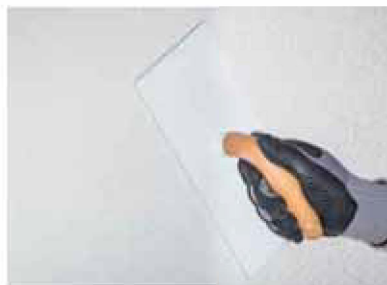
Figure 2 A plastic trowel is passed over the surface to form a texture before it dries.
