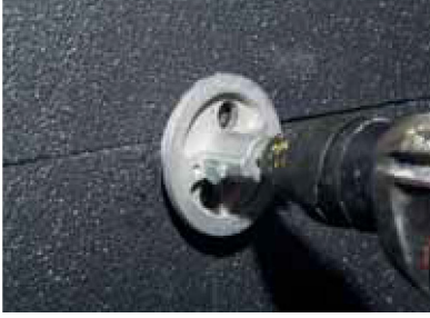
Figure 1 Counterboring by using apparatus is needed in order to place the wall plug head completely and to prevent thickness.
