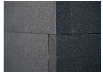
Figure 3 Thermal insulation boards are placed without gaps and in zigzag style upwards starting from the bottom of the wall. Boards should be placed in zigzag style on the corners as well.
