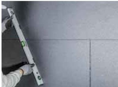
Figure 2 Board levels should be checked by straight edge or a water gauge.
