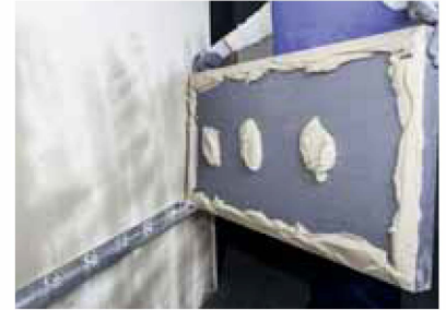
Figure 3 While applying adhesive mortar to the back of the insulation board, care is taken to prevent it from overflowing at the edges.
